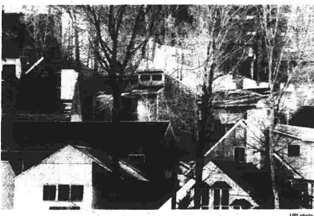
Another condominium takes shape in Sugarbush Village at Warren, Vt., recently. Resort development has come under fire by environmentalists and the Green Mountain State.
